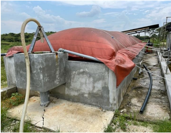
Methane fermenter and methane generator to generate electric from cattle waste
