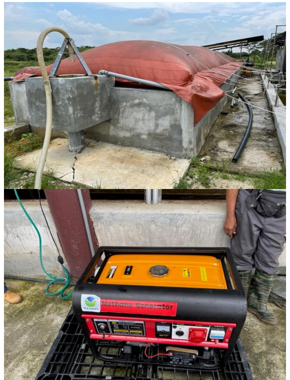
Methane fermenter and methane generator -Pusat Pertanian Moden, Kluang-
