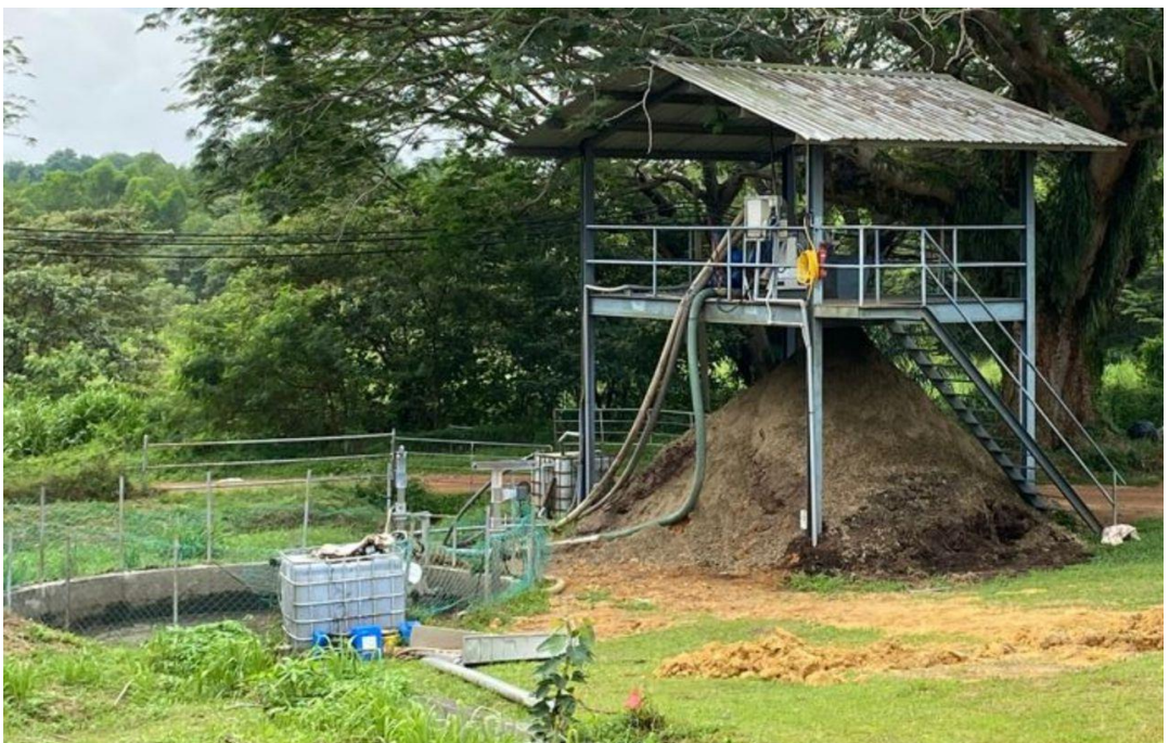
Cattle waste liquid and solid separation process. Solid waste used for bio-fertilizer. -Farm Fresh farm @ UPM-
