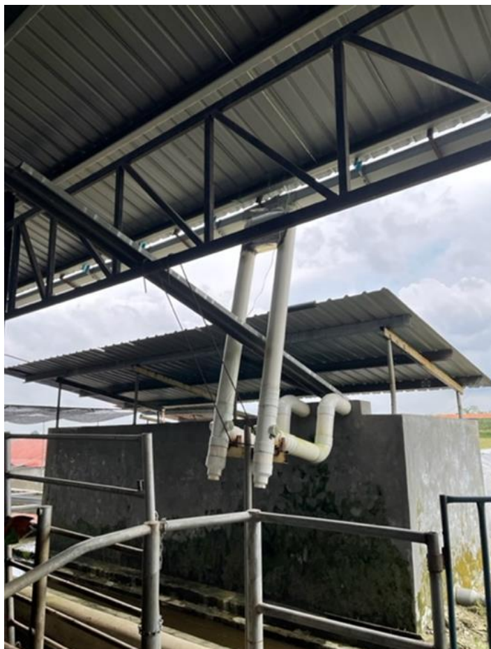
Rain water harvester tank -Pusat Pertanian Moden, Kluang-
